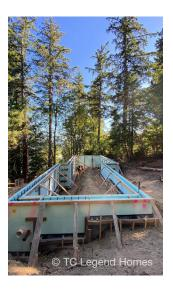
Insulated concrete foundations provide a well-insulated perimeter and require less labor than traditional forming.
