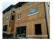
Two net-zero energy homes featuring structural insulated panels and triple-pane windows.
